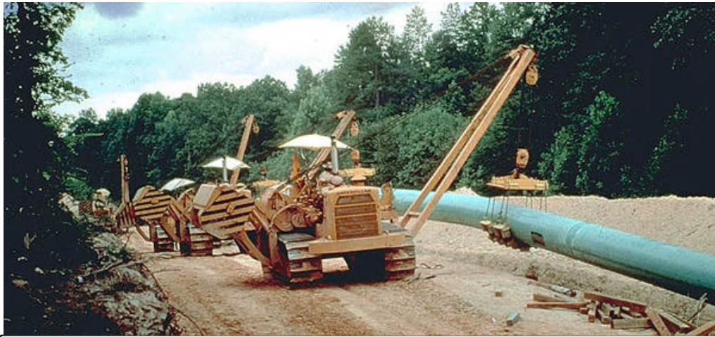
Figure 1. FBE pipeline coatings, in use since 1960, have been installed underground from equatorial desert sands to the arctic and in the ocean deeps.
