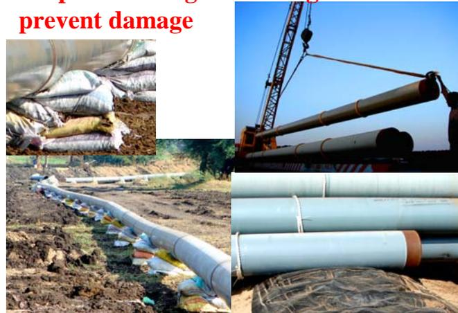
Figure 12: Use of plastic covered sand berms, sandbags, and padded hooks help prevent coating damage. Photos courtesy of J. A. Kehr.
