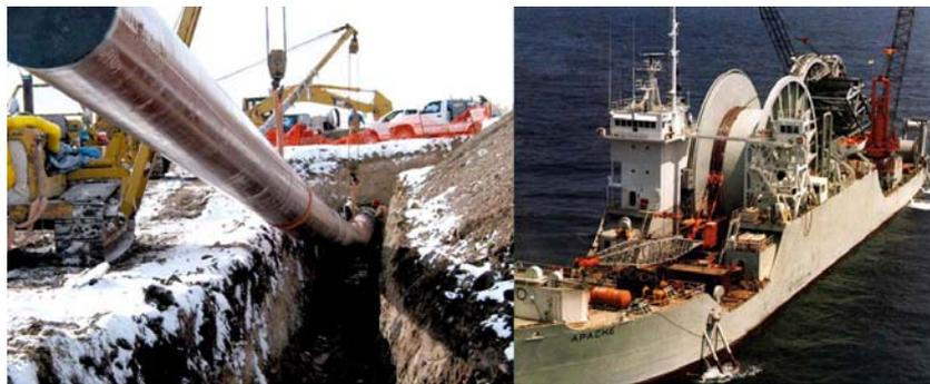
**Figure 18: Winter construction and reel-barge installation requires greater coating flexibility. Photos courtesy of M. Dabiri and Pipeline and Gas Journal.**
