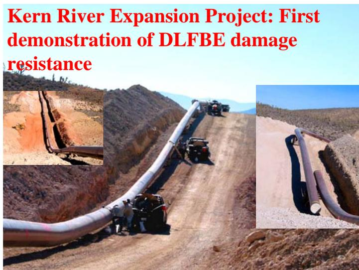
**Figure 10: The 1150 km 36" and 42" Kern River Expansion Project was the first to utilize DLFBE for the entire corrosion coating including girthwelds. Photos courtesy of M. Dabiri.**
