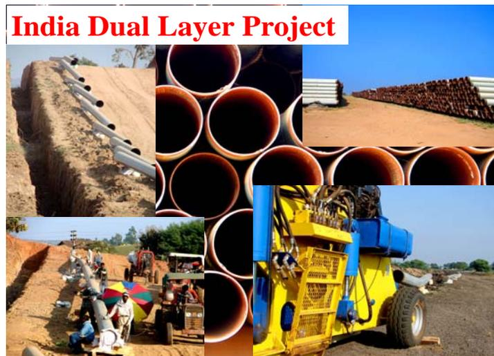
**Figure 9:** The Koyali-Ratlam Pipeline Project in India shows that a robust DLFBE coating system and well defined pipe handling guidelines can result in minimal coating damage even in areas with underdeveloped roads and infrastructure. Photos courtesy of J. A. Kehr.
